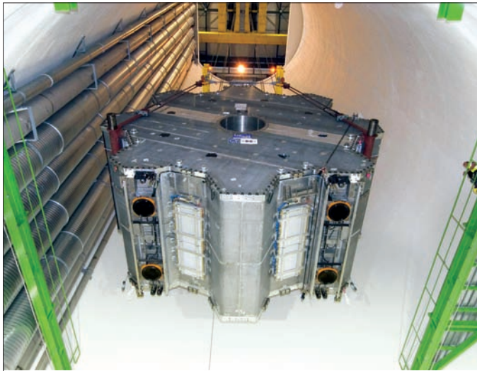
The first giant toroid magnet endcap on its 80 m journey to the floor of the cavern housing the ATLAS detector.
