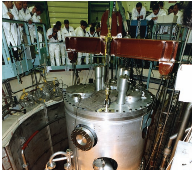
Installation of the new reactor vessel in February 1994 (ILL).
